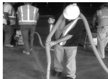
Example: New Construction joints being prepared using a vacuum
